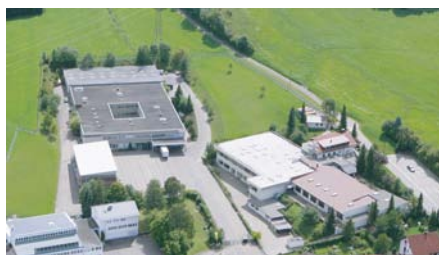
Firmenzentrale METZ CONNECT, Blumberg
